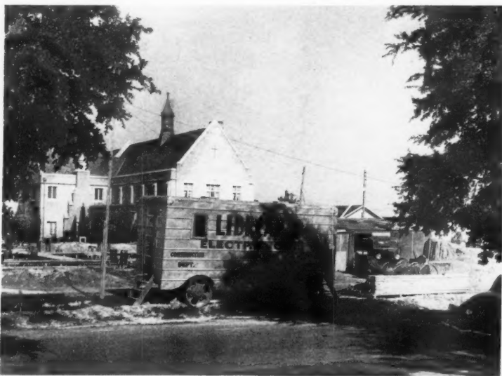
This portable field office operated by the Libecap Company contains office records and blueprints as well as special tools.
